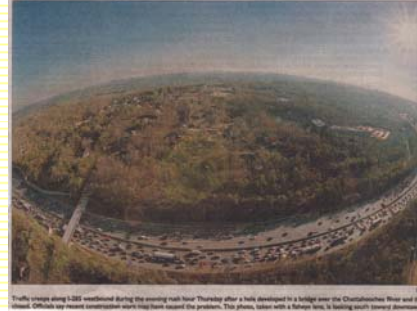
Traffic snarls along I-285 ventilation during the evening rush hour Thursday after a hole developed in a bridge over the Chattahoochee River and it closed. Officials say recent construction work may have caused the problem. This photo, taken with a fisheye lens, is looking south toward downtown Atlanta.
